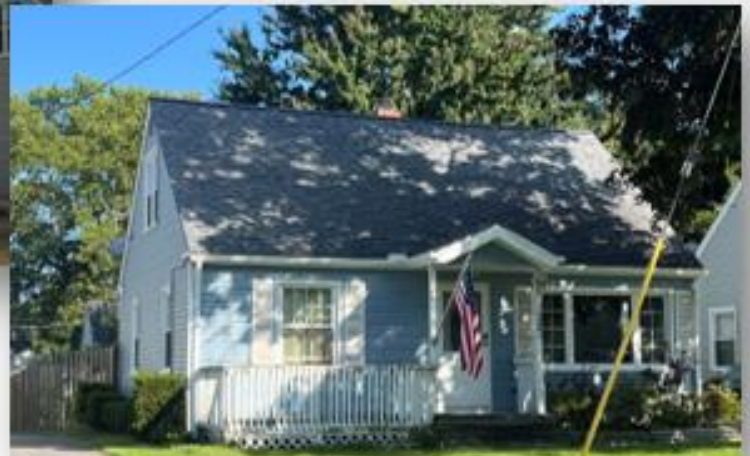
1221 Crescent Drive: Siding After
