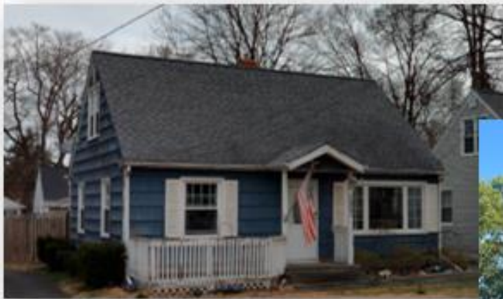
1221 Crescent Drive: Siding Before
